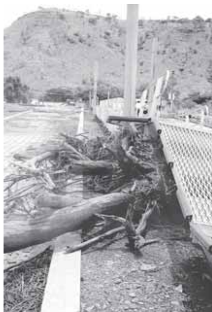
Unsuitable: A new $6m public jetty has been proposed for Wyndham. Residents say the current jetty (pictured here: showing recent damage caused by floating Gulf debris) is not safe for cruise ship passengers wanting to alight in the town.
